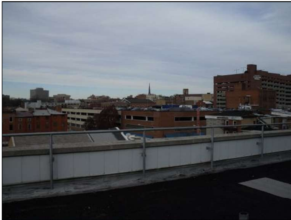
Roof B-Overview, looking North
