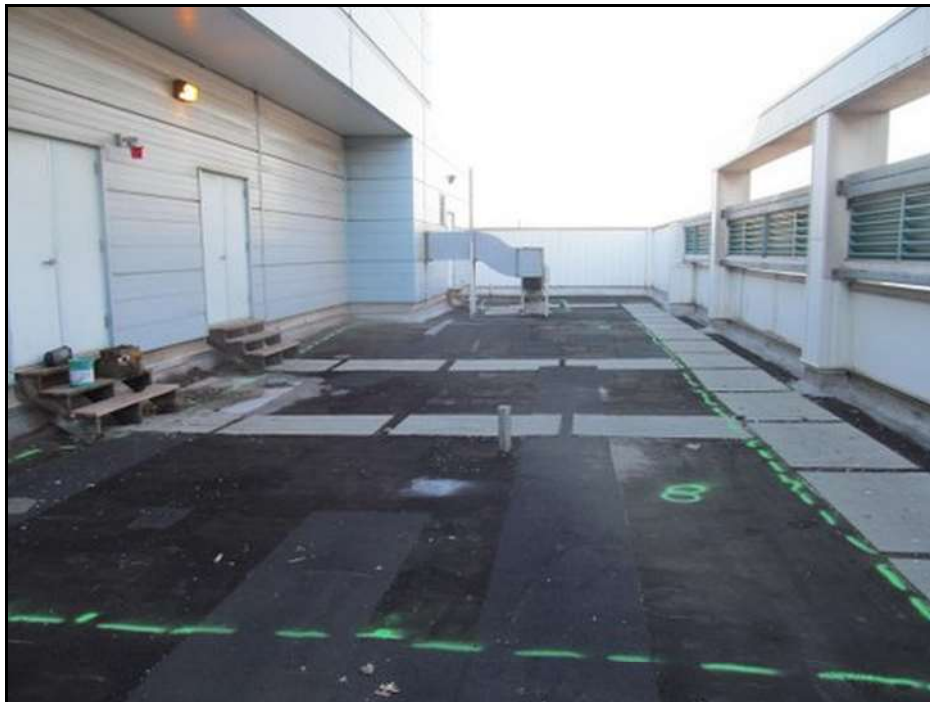
Roof A-Wet Area 8, looking North. This wet area was found using a Capacitance DEC Scanner and therefore there is no thermal image available.
