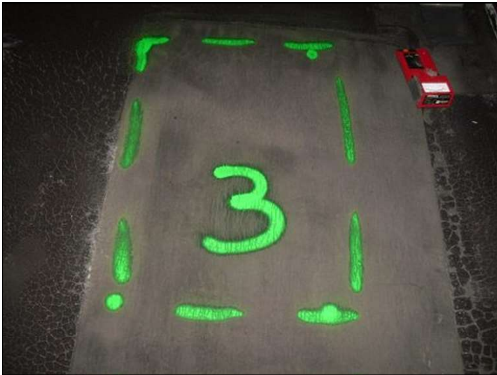
Roof G-Wet Area #3, looking West
