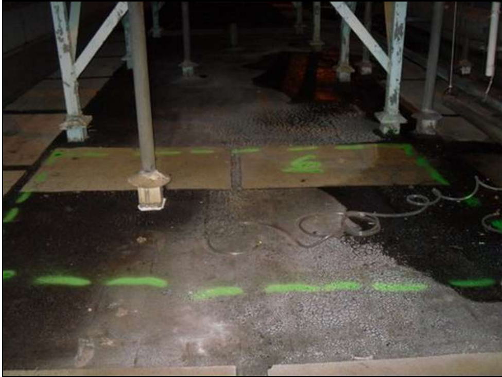
Roof A-Wet Area #6, looking North
