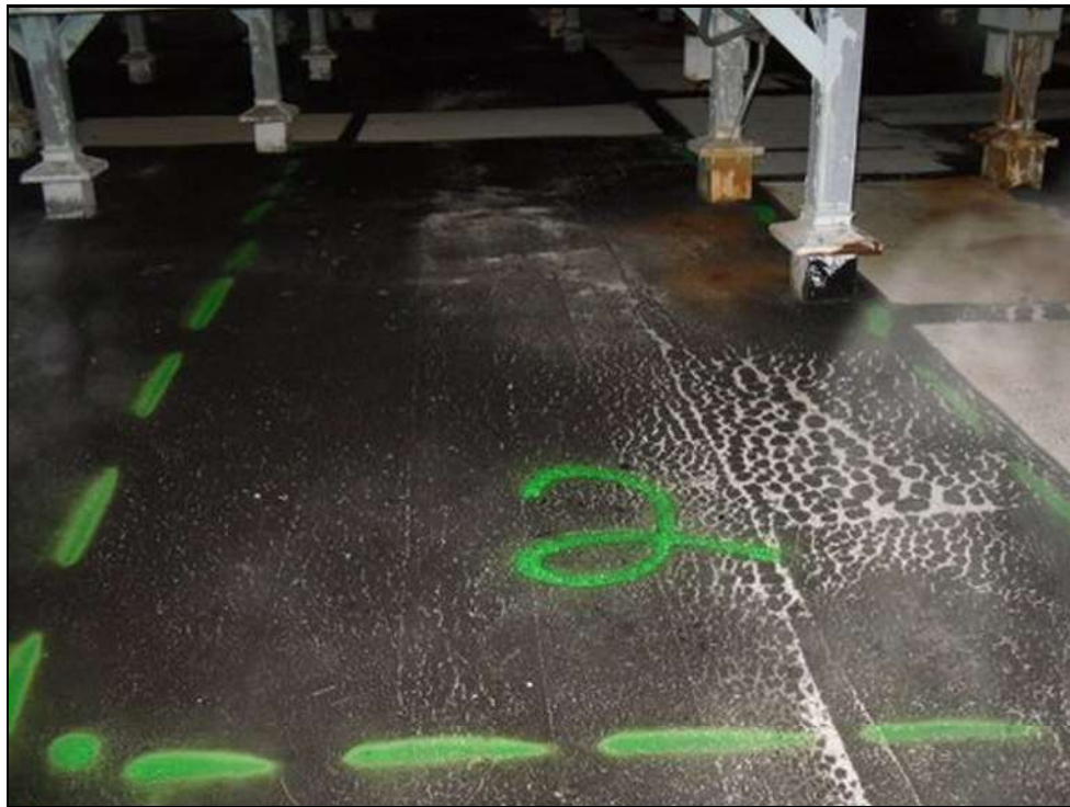
Roof C-Wet Area #2, looking South
