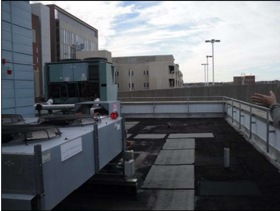
Roof B-Overview, looking West
