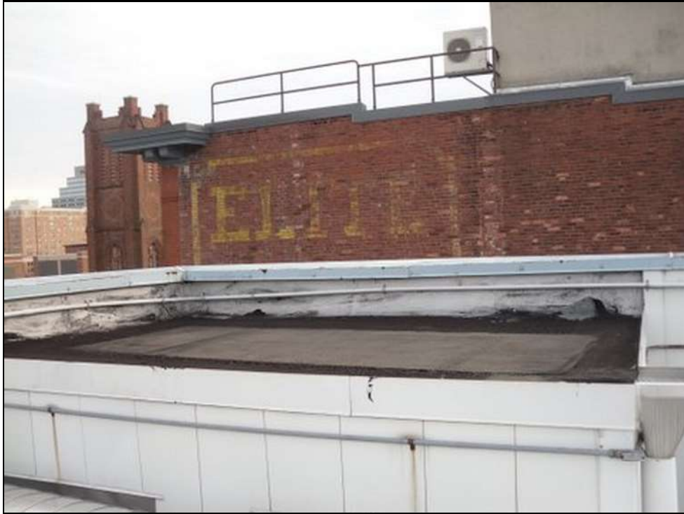
Roof G-Overview, looking South
