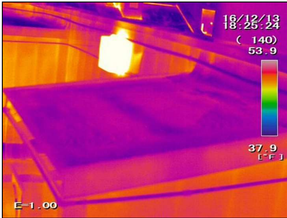
Roof H-Overview, looking East. No thermal anomalies, consistent with moisture intrusion, were noted.
