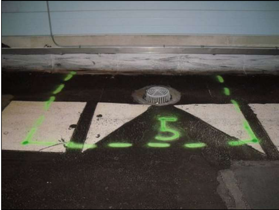
Roof A-Wet Area #5, looking East
