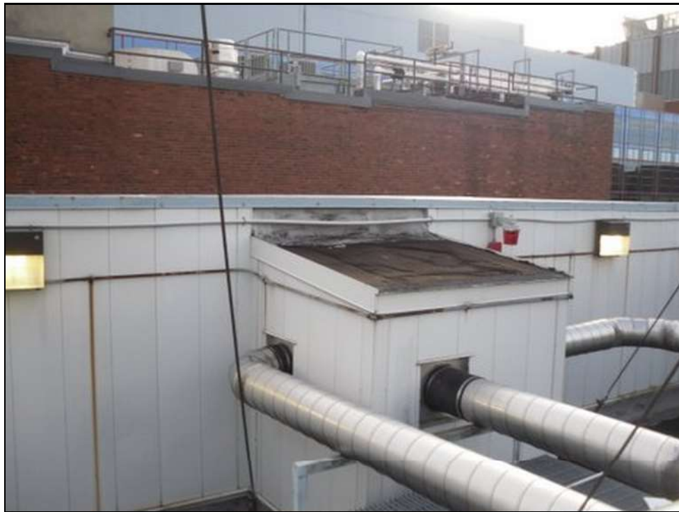
Roof H-Overview, looking South
