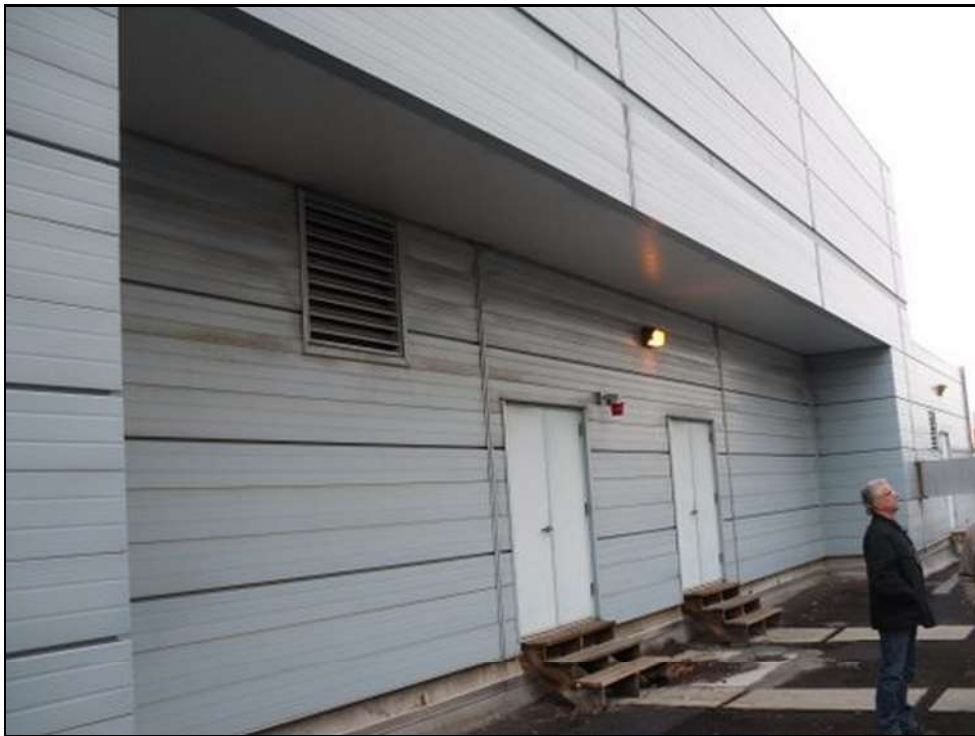
Roof A-Overview, looking West
