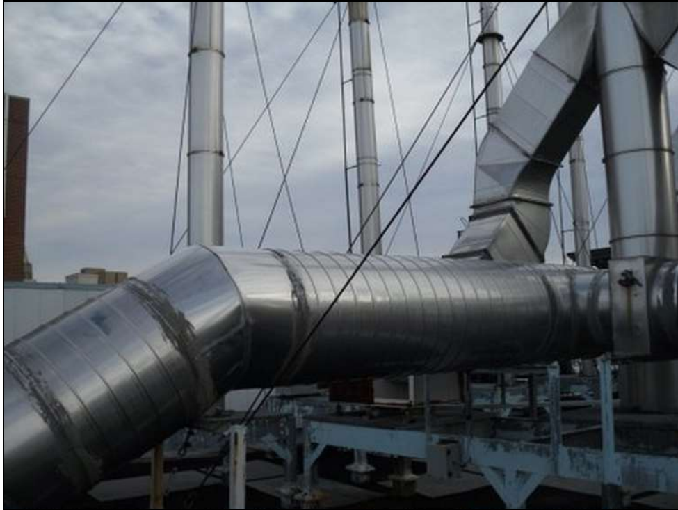
Roof C-Overview, looking East
