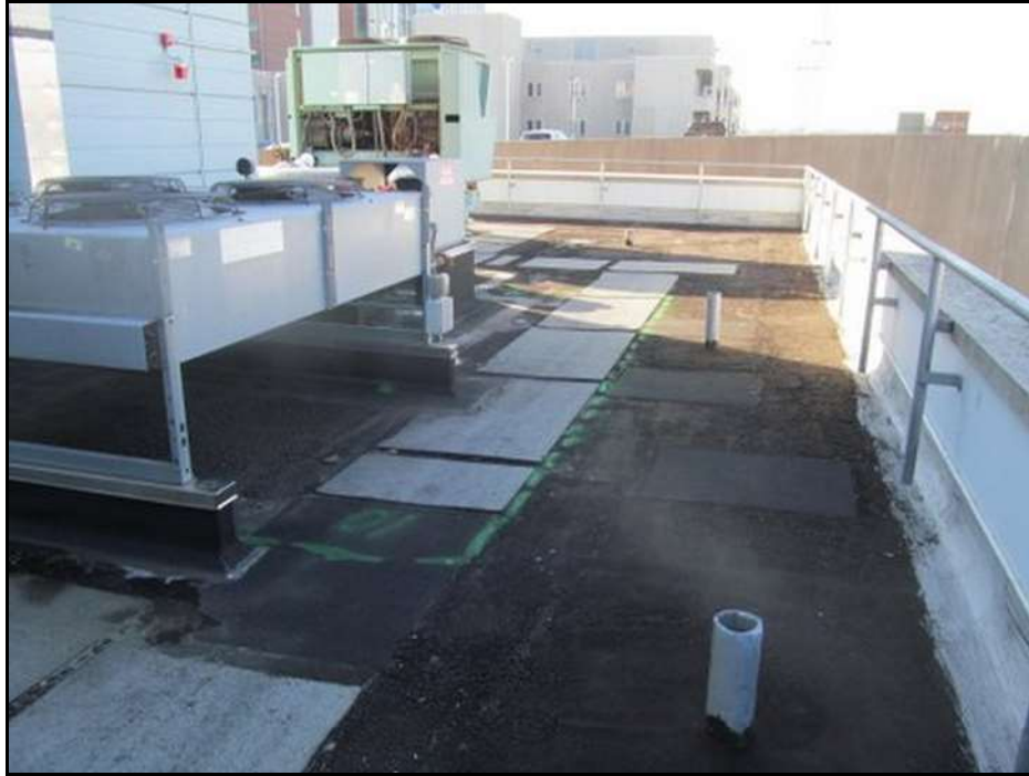
Roof B-Wet Area #10, looking West. This wet area was found using a Capacitance DEC Scanner and therefore there is no thermal image available.
