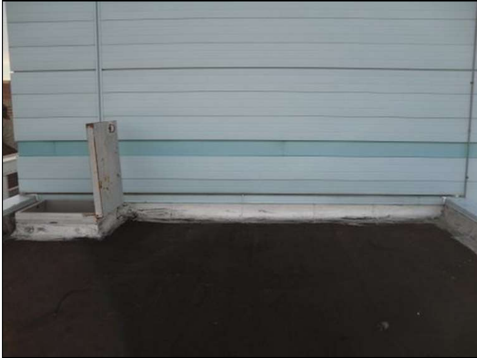
Roof D-Overview, looking South
