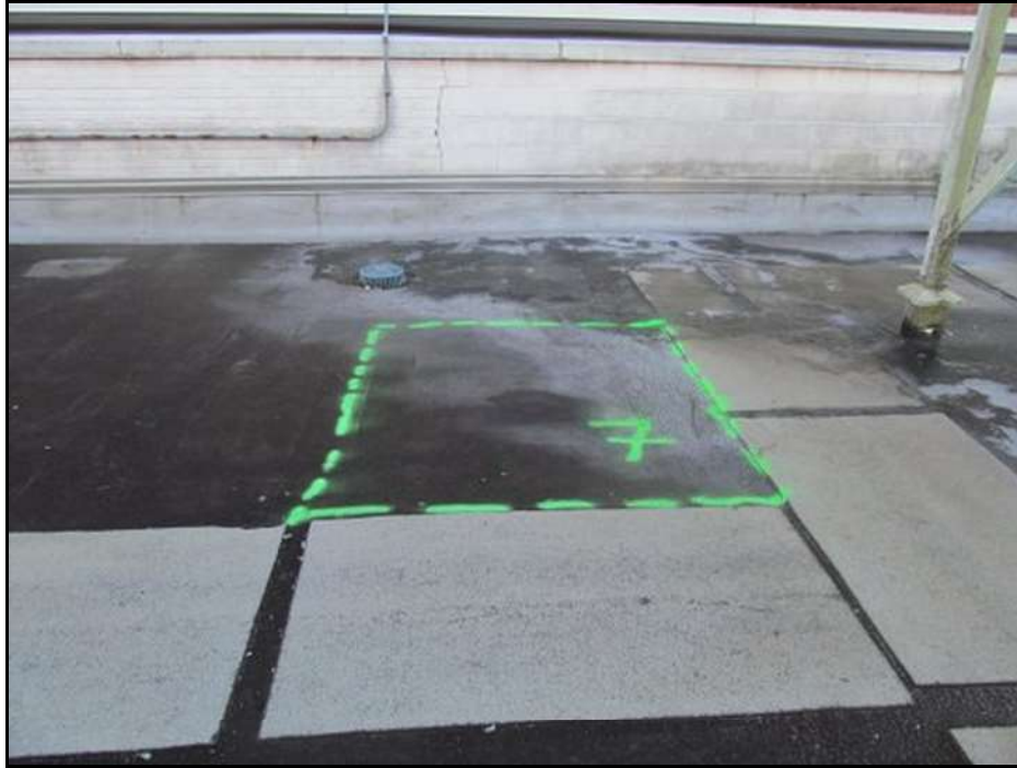
Roof A-Wet Area #7, looking South. This wet area was found using a Capacitance DEC Scanner and therefore there is no thermal image available.
