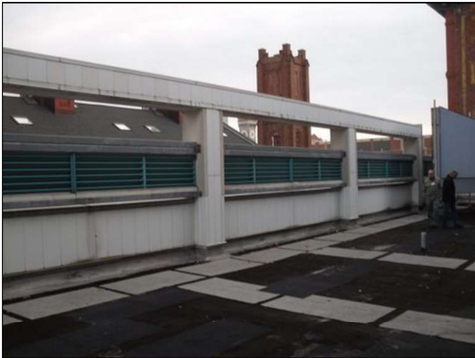
Roof A-Overview, looking East
