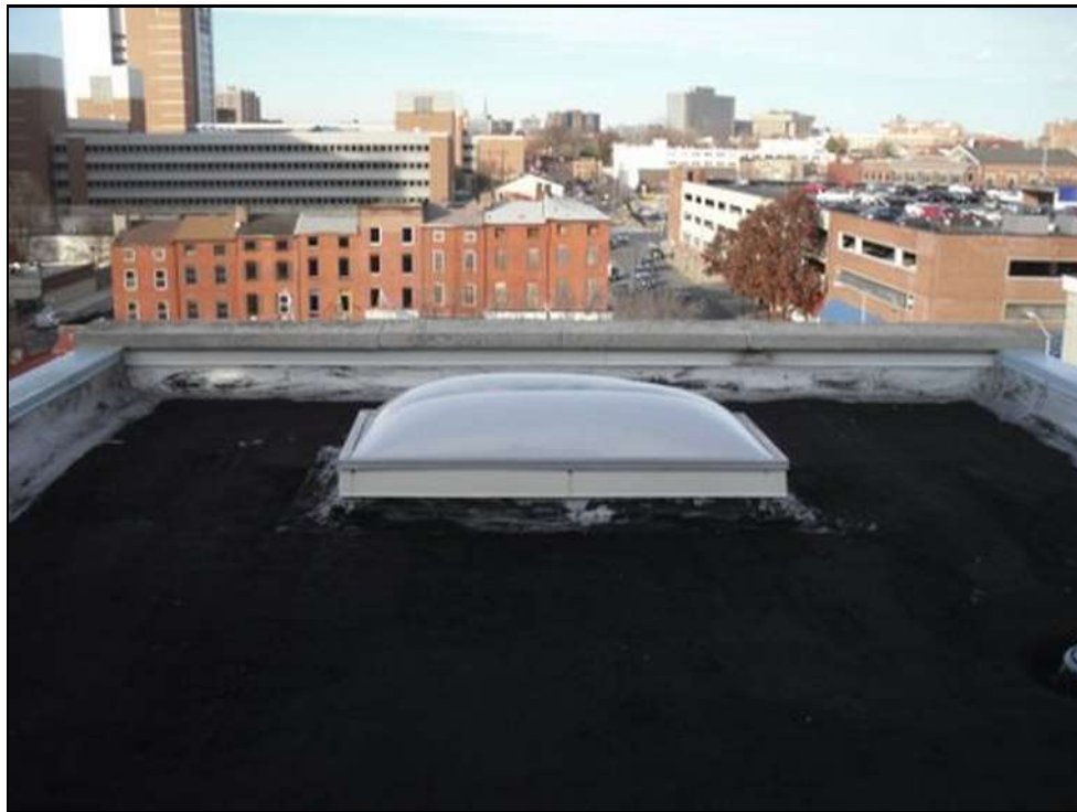
Roof D-Overview, looking North
