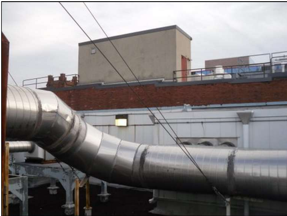
Roof C-Overview, looking South
