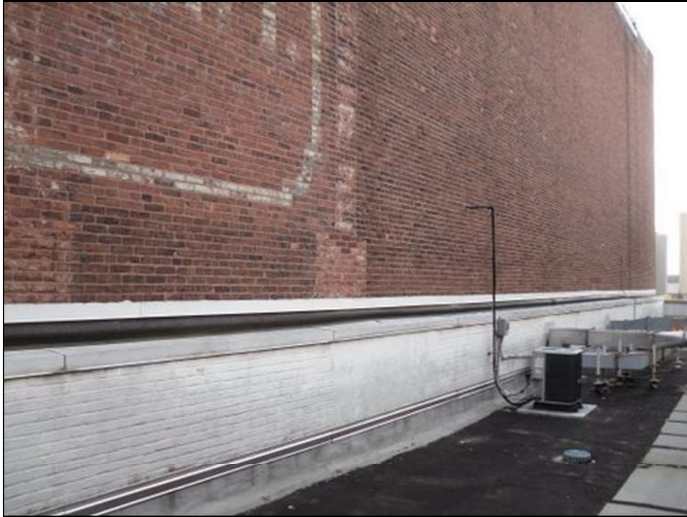
Roof A-Overview, looking South
