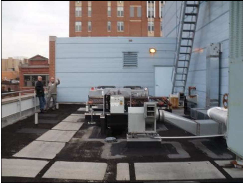
Roof B-Overview, looking East
