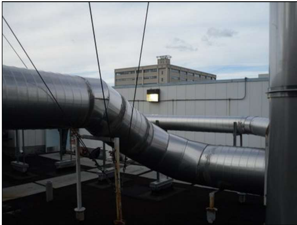
Roof C-Overview, looking North
