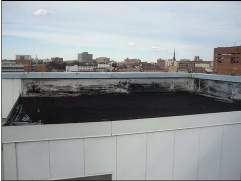
Roof F-Overview, looking North
