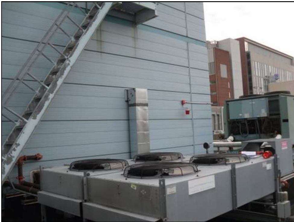
Roof B-Overview, looking South
