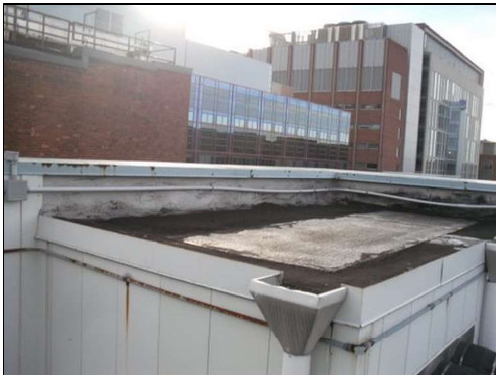
Roof I-Overview, looking South
