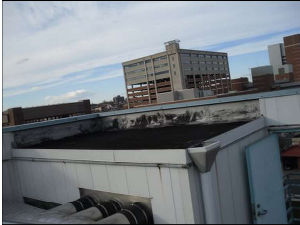
Roof E-Overview, looking North
