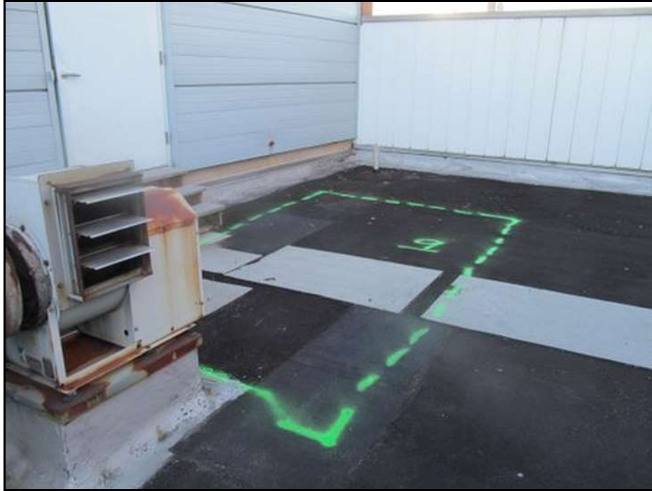
Roof A-Wet Area #9, looking North. This wet area was found using a Capacitance DEC Scanner and therefore there is no thermal image available.
