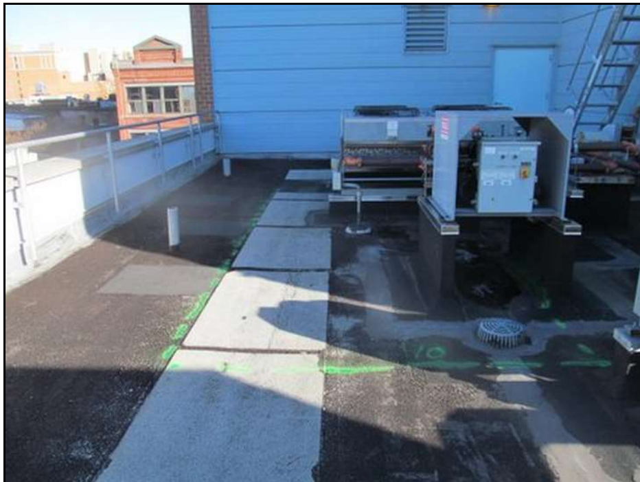
Roof B-Wet Area #10, looking East. This wet area was found using a Capacitance DEC Scanner and therefore there is no thermal image available.
