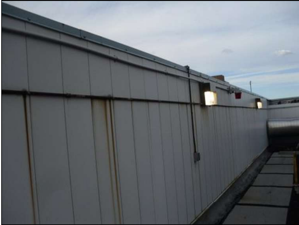
Roof C-Overview, looking West
