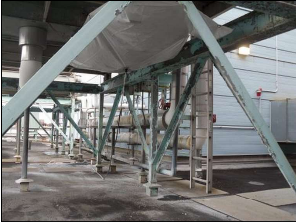
Roof A-Overview, looking North
